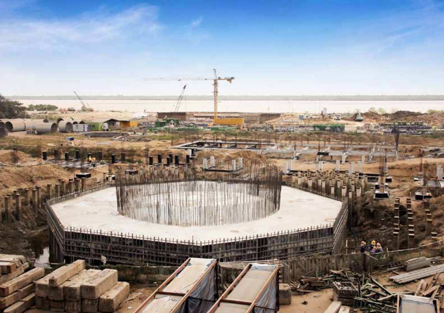
Long Phu 1 Thermal Power Plant - Main contractor for foundation of chimney structure
