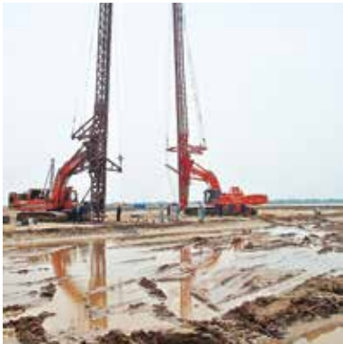
LG Display Vietnam Hai Phong - Soil improvement by PVD installation & DCM method: 50,234m
