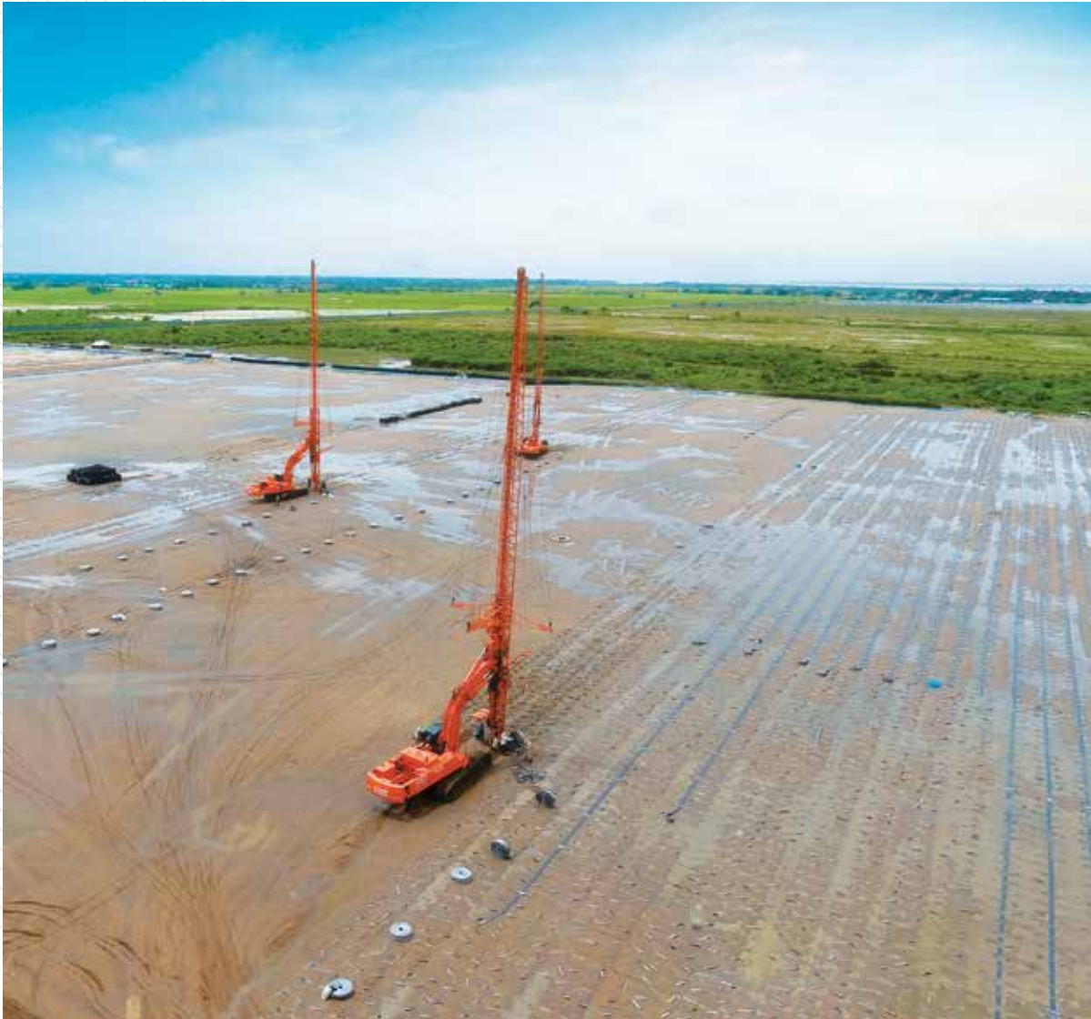
Thilawa Port (Myanmar) expansion - Soil improvement in PVD method
