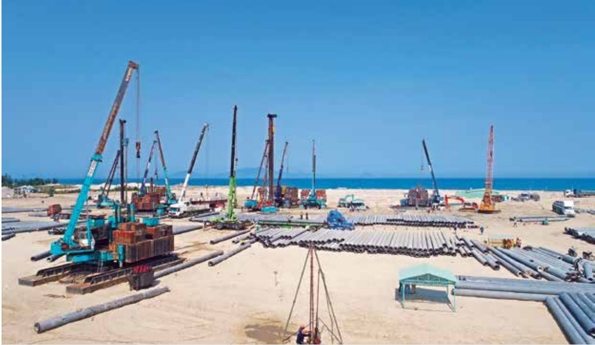
Hoiana Hotel & Casino Complex - Supply & installation of PHC pile D350, D500; Pre-boring works
