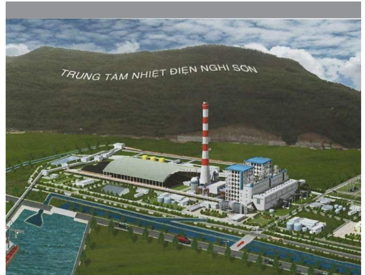
Nghi Son 1 Thermal Power Plant
