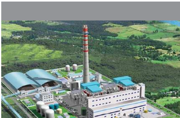
Thai Binh 1 Thermal Power Plant
