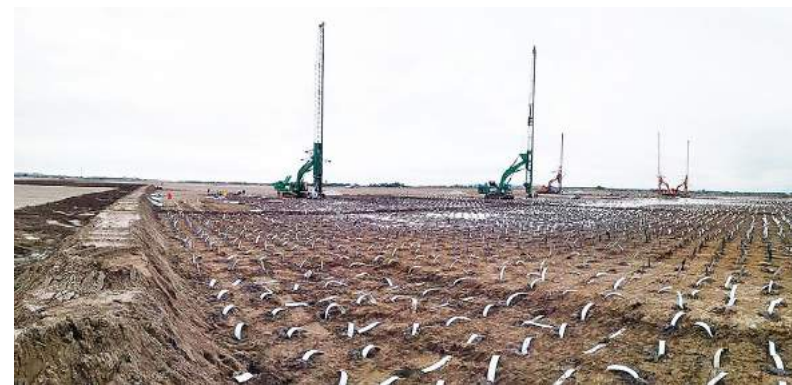
Flat PV Glass Factory Supply and PVD installation, Sand pre-loading.
