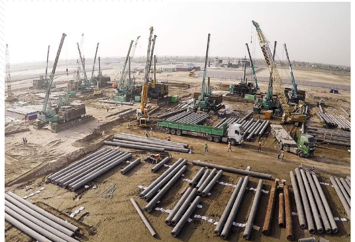
Piling works at Thai Binh Thermal Power Project
