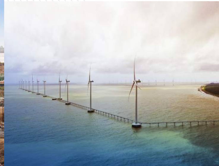
Tra Vinh V1.3 Wind Power Plant Project
