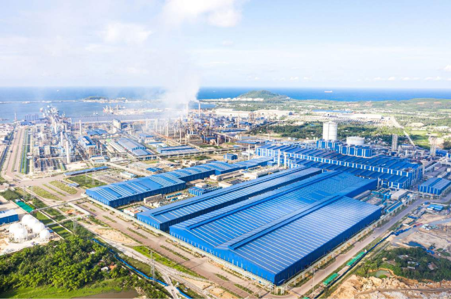
Hoa Phat – Dung Quat Steel Factory Project
