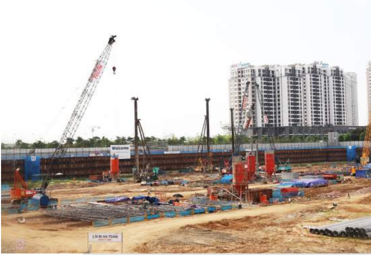
Lotte Mall (Hanoi) Project
