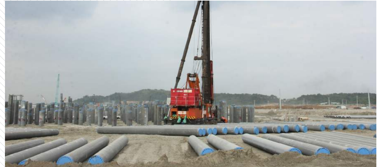
Piling works at Long Son petrochemical refinery project
