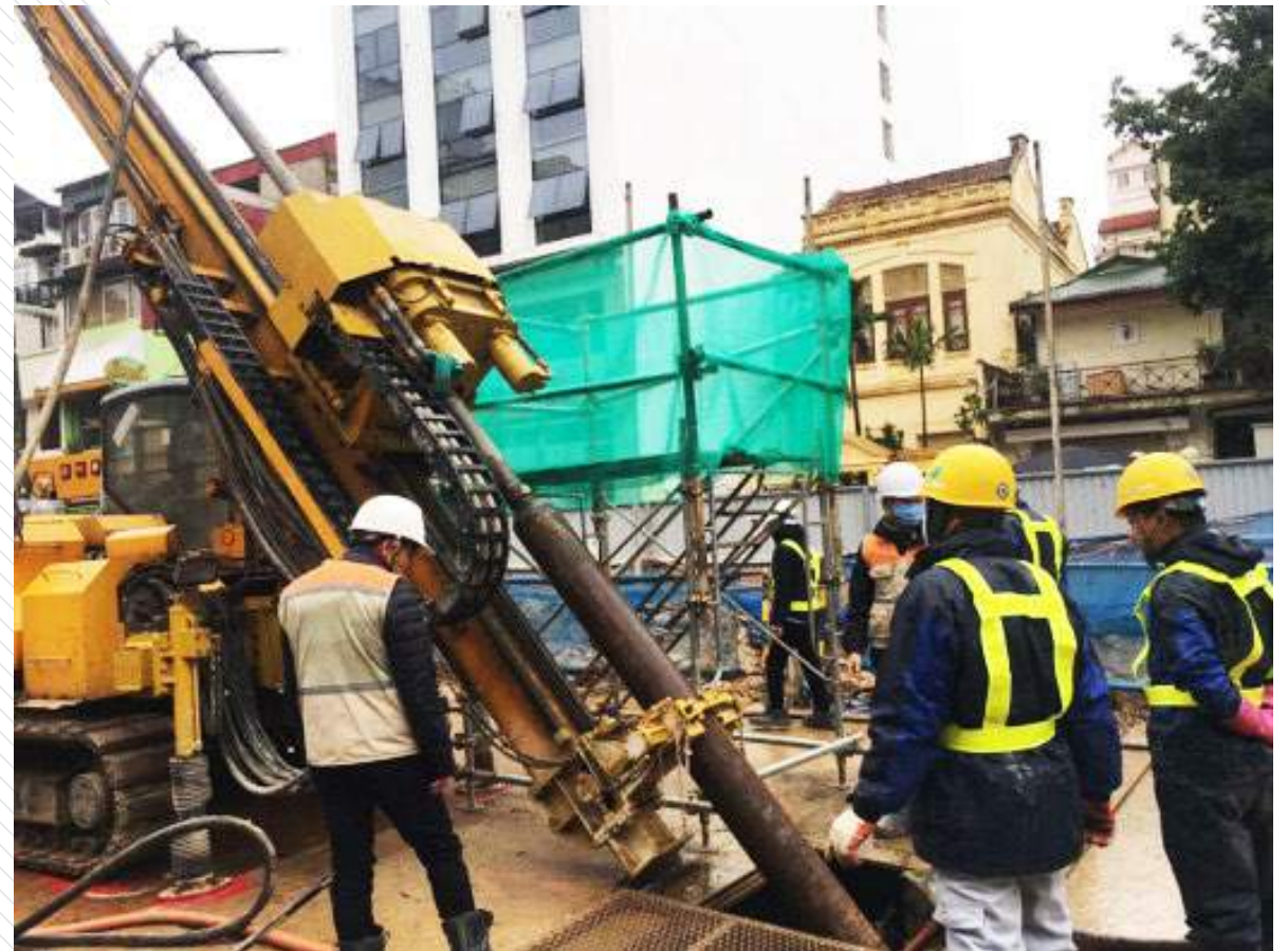
3 Pic 3. Metro Line 3 (Hanoi) Jet Grouting technology
