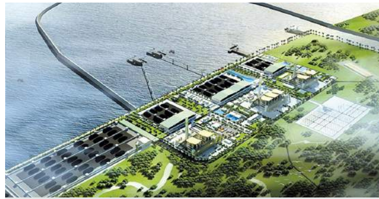
Expanded Duyen Hai 3 Thermal Power Plant
