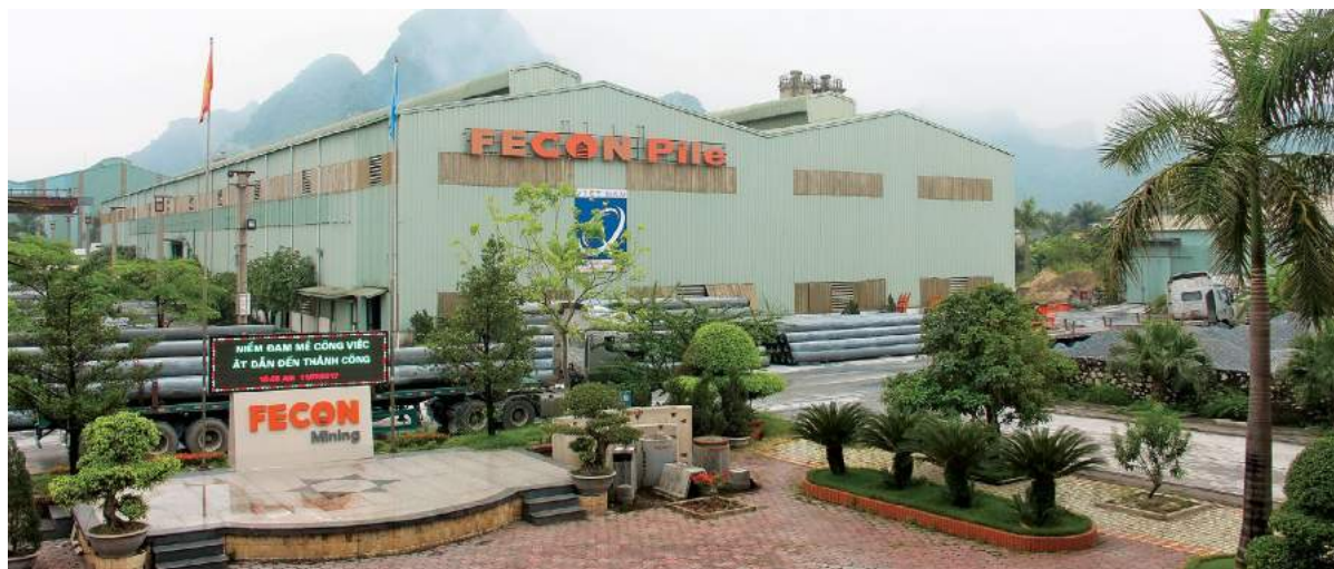
FECON Pile Factory in Ha Nam
