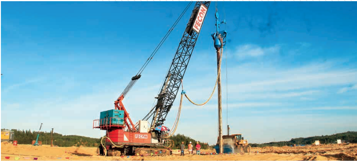
Hoa Phat (Dung Quat) Steel Factory - Vibro compaction and vibro replacement
