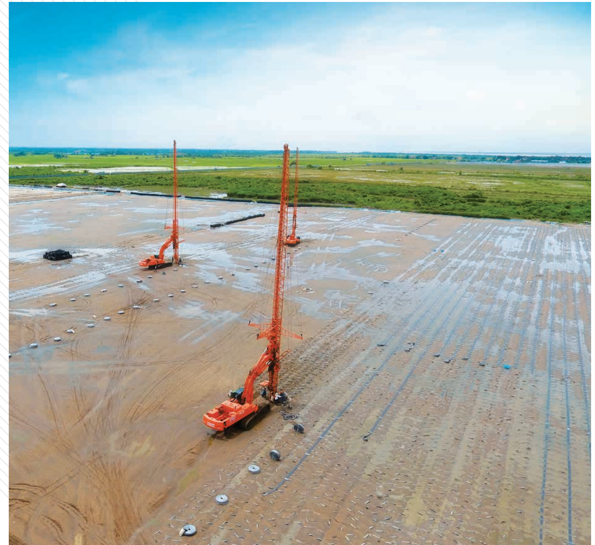
Thilawa Port (Myanmar) expansion - Soil improvement in PVD method
