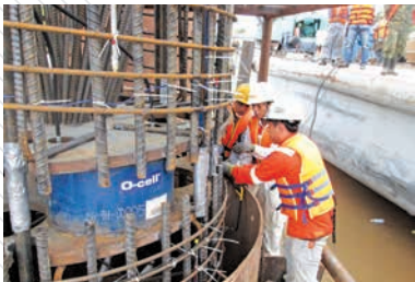
Cao Lanh Bridge - O-Cell load test for bored pile with diameter of 2500mm
